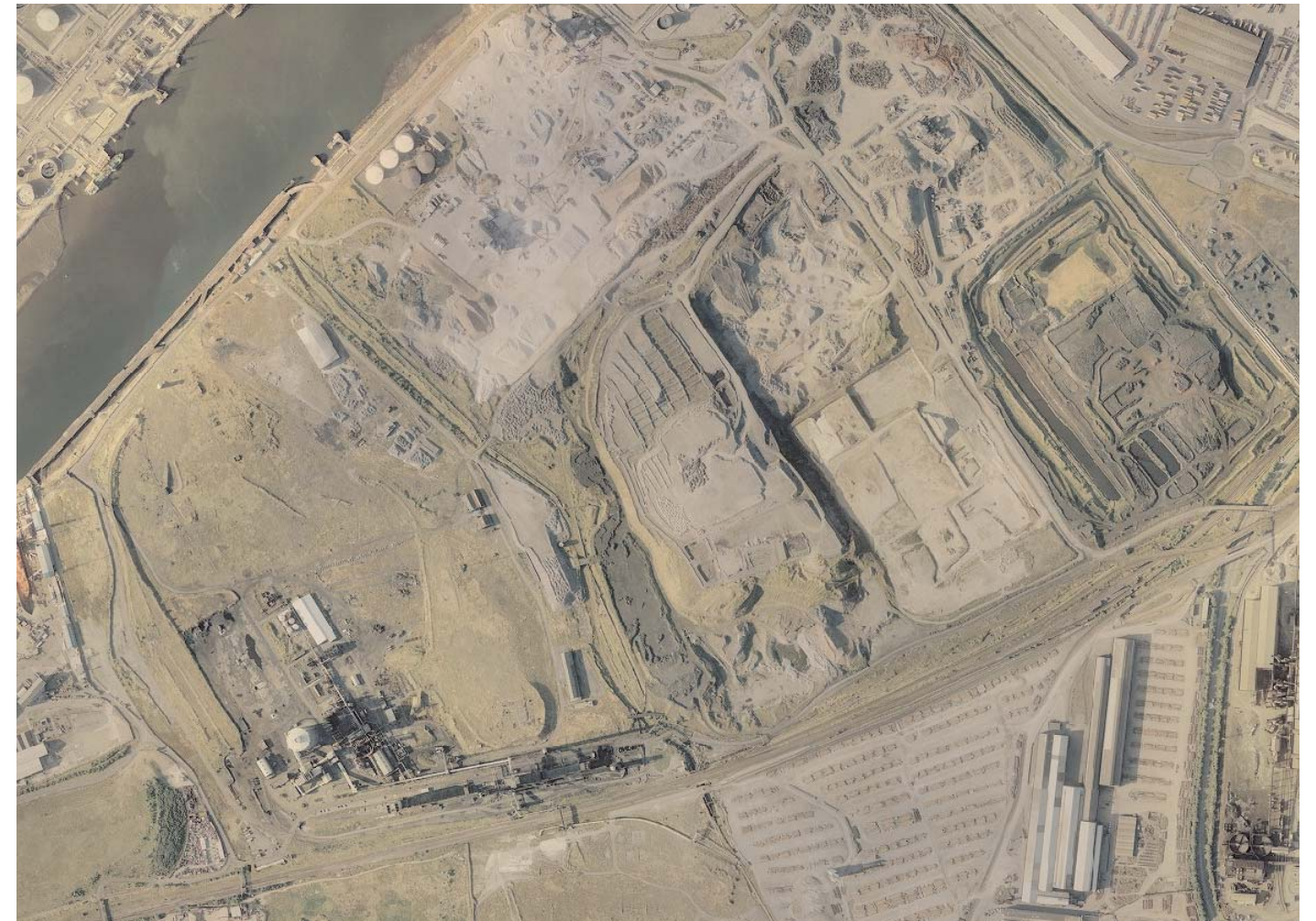
Aerial Photo - Cleveland
