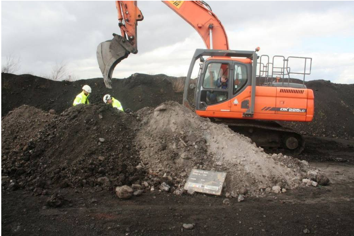
Figure TP106.3 TP106 - Trial Pit Spoil
