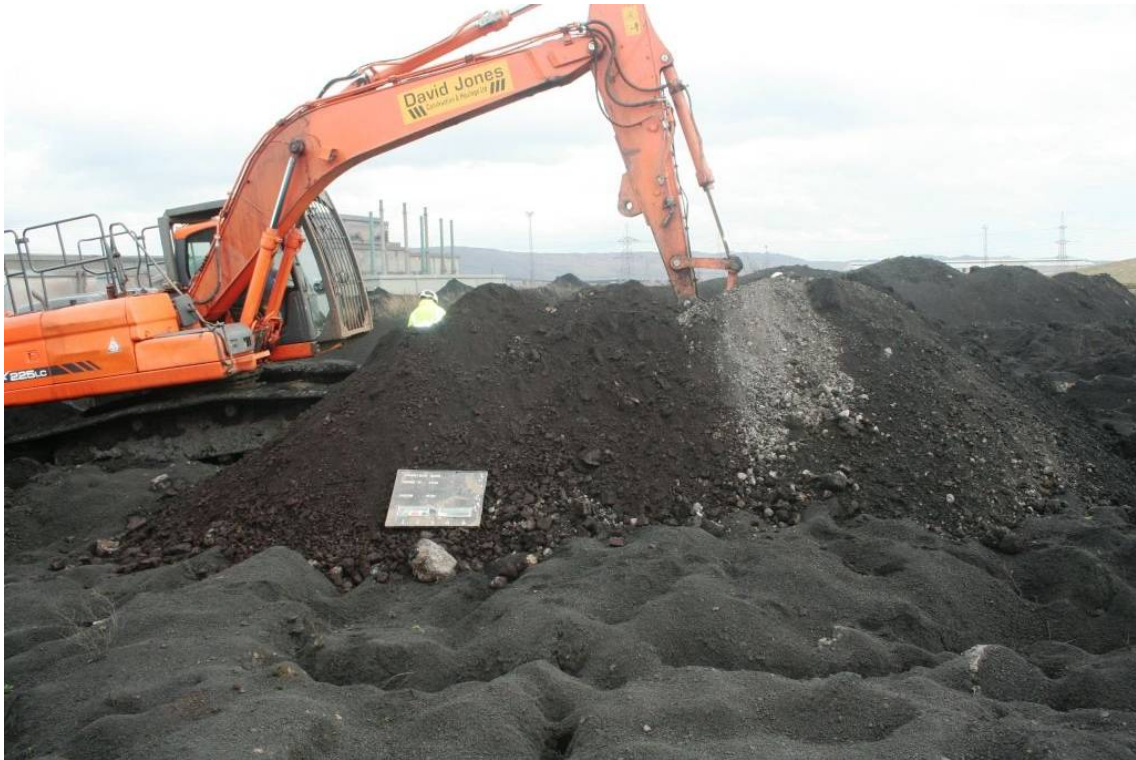
Figure TP104.3 TP104 - Trial Pit Spoil
