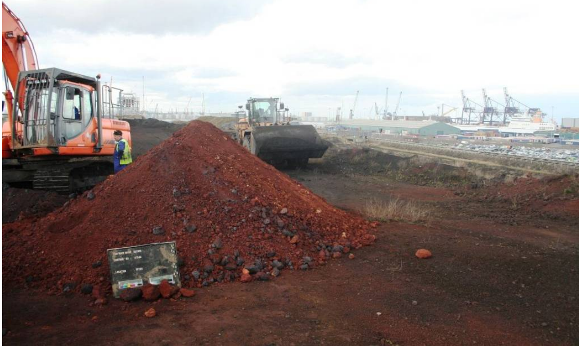
Figure TP105.3 TP105 - Trial Pit Spoil
