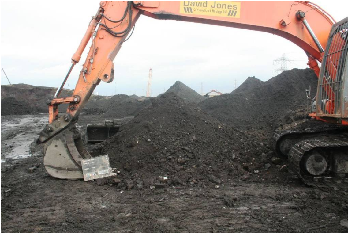
Figure TP108.3 TP108 - Trial Pit Spoil
