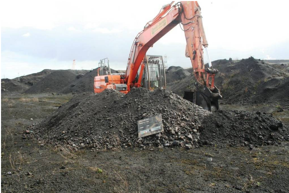
Figure TP101.3 TP101 - Trial Pit Spoil
